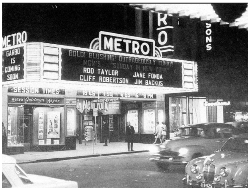
Figura 1 - Cinema Metro, Hindley Street; Adelaide (1964)
